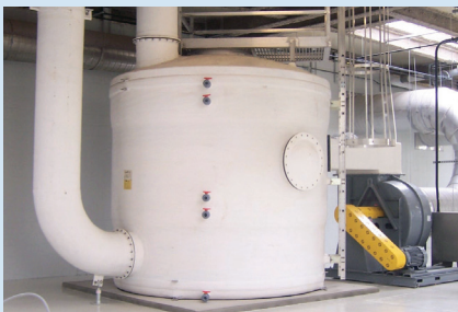
VESSEL SCRUBBER Large headworks, full treatment plants, and digesters 8,000 - 20,000 CFM
